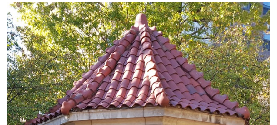
Historic clay tile roof
