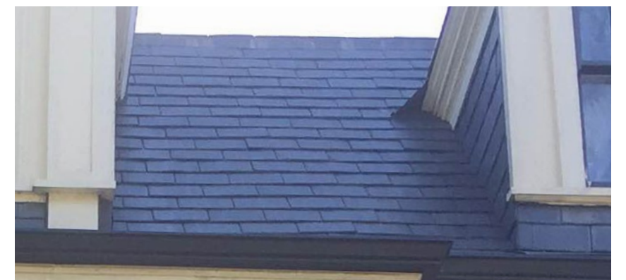
Asphalt shingle roof
